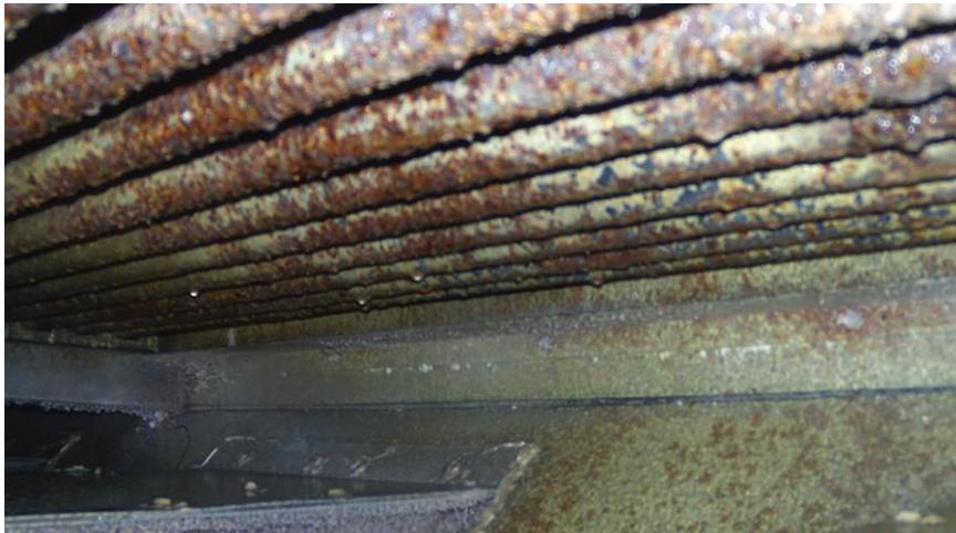
When water is heated or evaporated, scale often is left behind. Scale can affect the efficiency of water-cooled systems and the overall equipment longevity.
